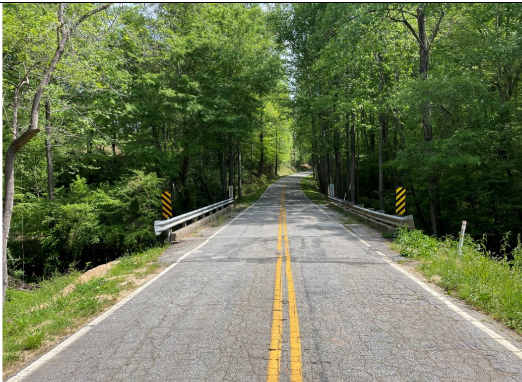
Photograph 10 – S-226 Bridge Facing Northeast
