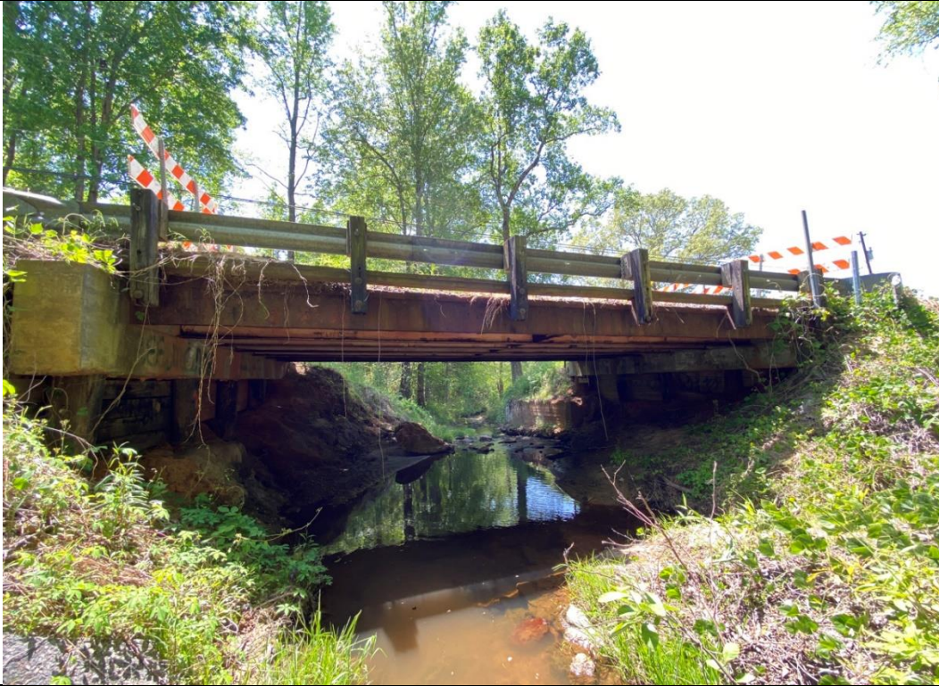
Photograph 7 – S-106 Bridge and Suck Creek Facing South
