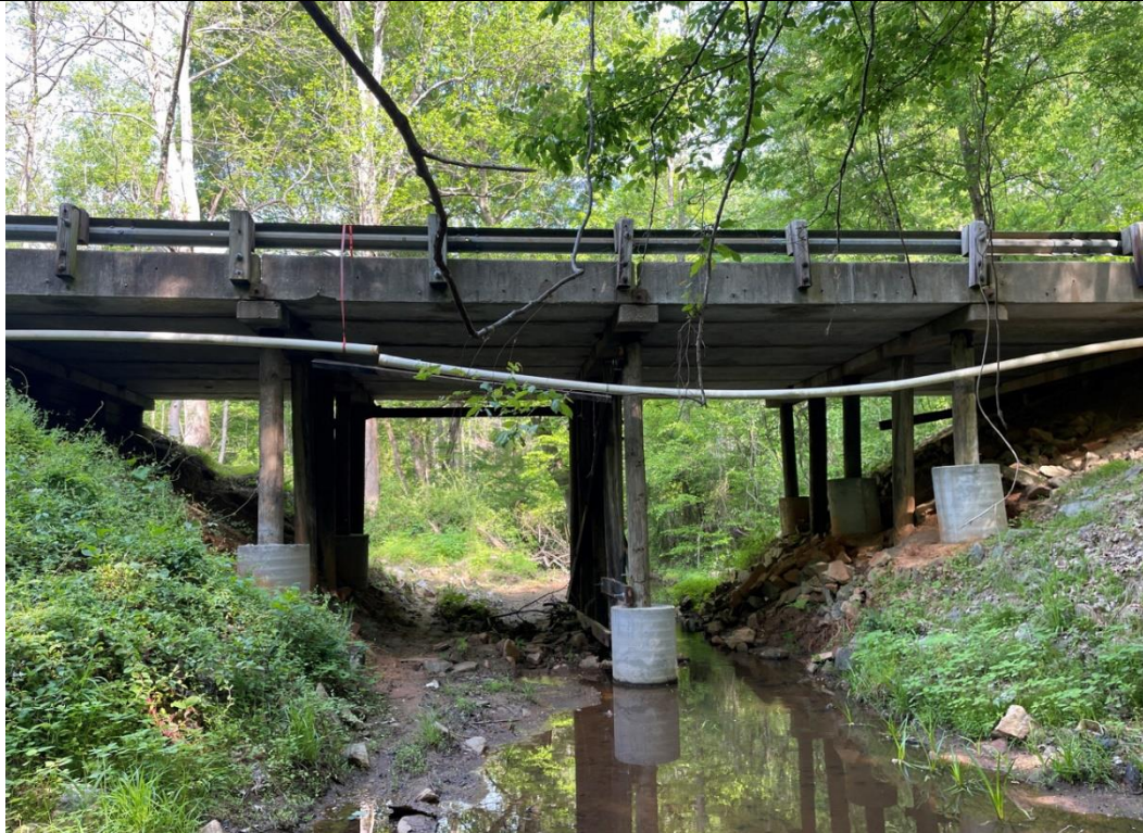
Photograph 9 – S-226 Bridge and Hammett Grove Branch Facing Northwest
