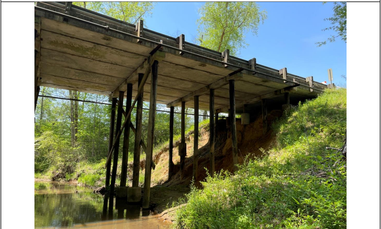
Photograph 8 – Bridge at Goucher Creek Facing West
