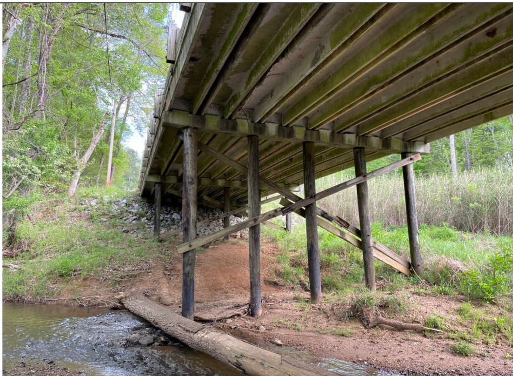
Photograph 8 – Bridge at Kings Creek Facing South
